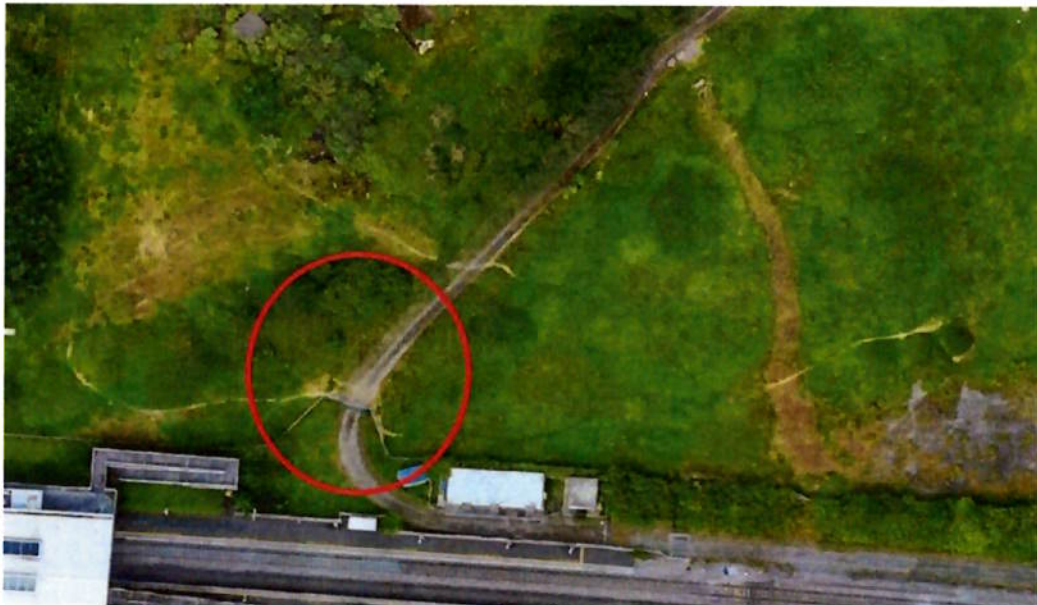
Access Gate Location
